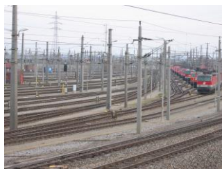
Marshalling Yard Kledering
