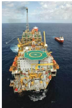
FPSO CARATINGA Petrobras P48
